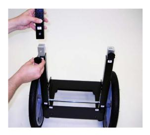
**9.** Locate and install two (2) of the 3/8-16 Short thumb screws into the back of the bottom uprights, tightening the two sections of the uprights together. Once you have done this, your cart should look like the photo below:
